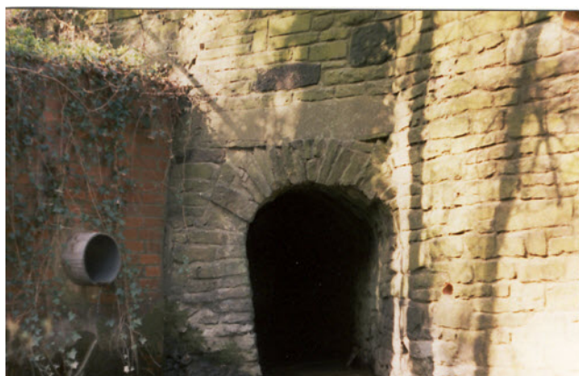
Franktonhook Bridge in the dip below The Fox Inn had to be built over the ravine carrying a convergence of two streams down to the Arun. The wing walls are clearly later reinforcements, but here on the south side of the culvert is the original facing wall with its stout stonework and arch ring as set by the contractors to the Turnpike Trustees. Rural bridges were only of single cart's width, and the interior stonework reveals that it was widened twice on the north side. The first was possibly in 1891 when delegates of the Vestry met with the parish surveyor to discuss its widening and repair, and a further widening was with shuttered concrete which unlike the older stonework has settled and cracked. This was possibly done in 1941 when a length of road on the north side was widened at Bucks Green.
