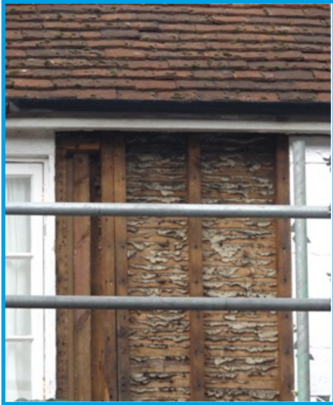
Example of a lath and plaster wall
